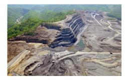
Dig expansive trenches to remove *overburden*, then fill with loose rock in *spoil bank*s
